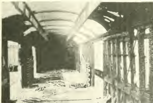
Interior of Wooden Car after Fire.
